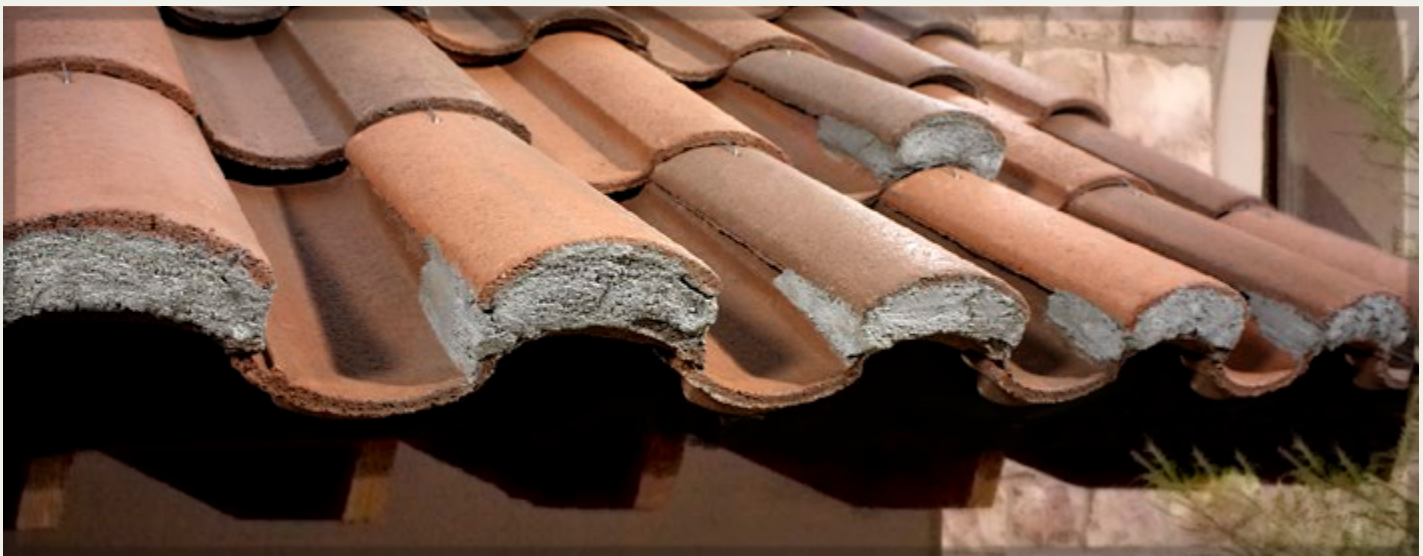
Close-Up of Boosted Eave
